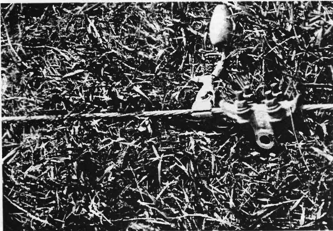
Fig. 1-6 (b) : Shield wire after separation from static mast
